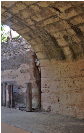
Detail view of west bridge wall at the trail, showing overpaint treatment of graffiti and moisture migration through the upper vault mortar joints.
