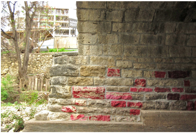
At Location 2 and 3, the coated stones remain discolored, even after the completion of the graffiti removal work.
