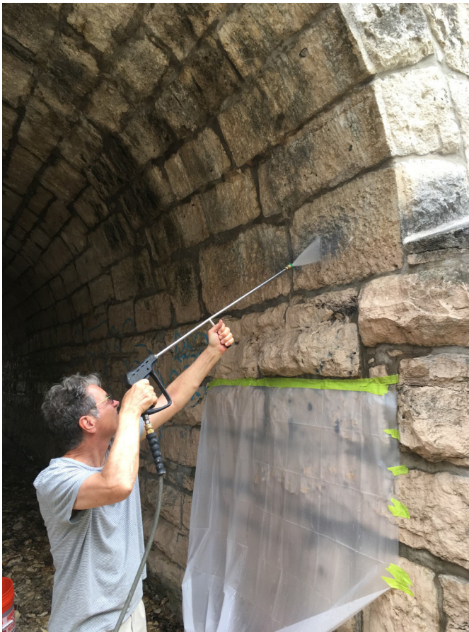
The graffiti was removed with a high-pressure cold water washer, using municipal water.
