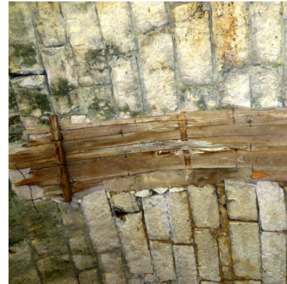
Utilities cut into arch stones
