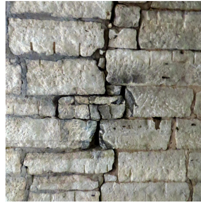
Broken stone / Missing mortar
