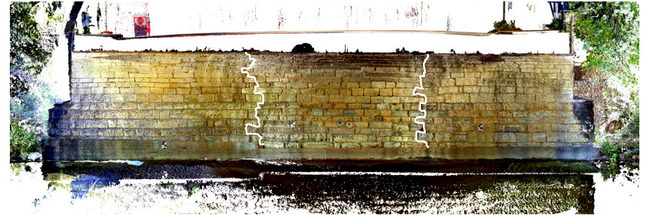
West Sixth Street Bridge, middle vault longitudinal section showing construction joints within the length.
