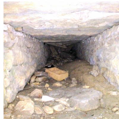
Tunnel collapse, vault A
