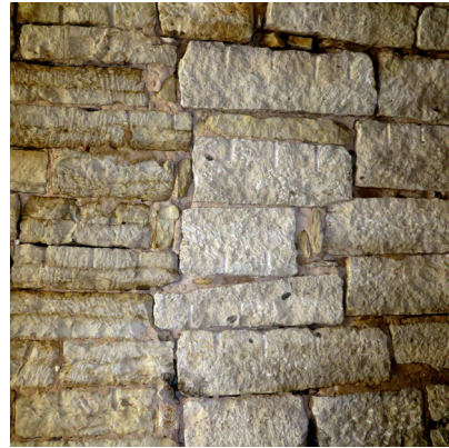
Construction joint - change in stone -
